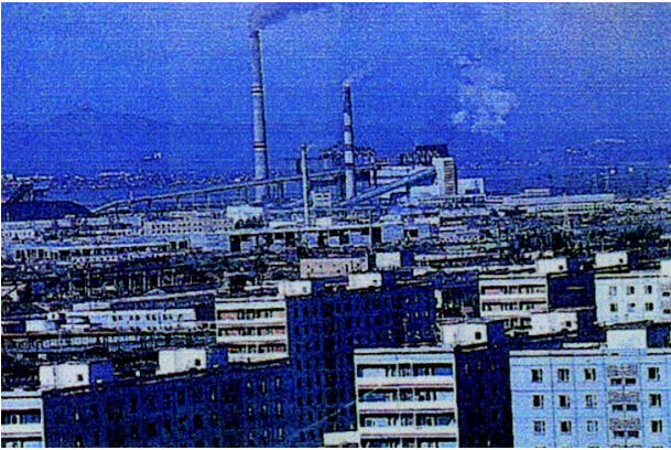
Photo 3.4 Emissions from thermal power plant in Ulaanbaatar
