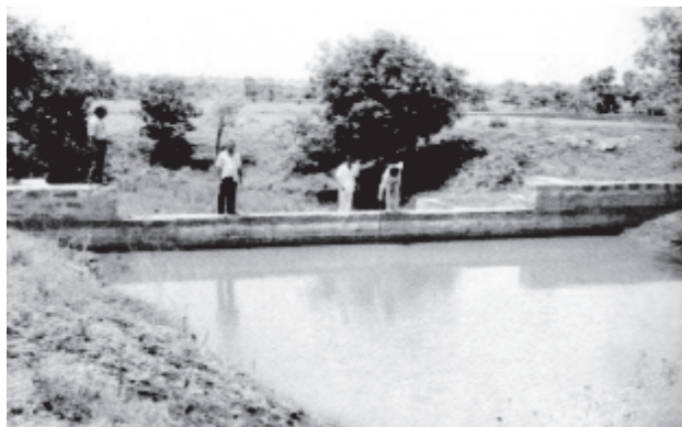
Photo 11.5 Masonry gully control structure having harvested water in Parua Nala watershed
