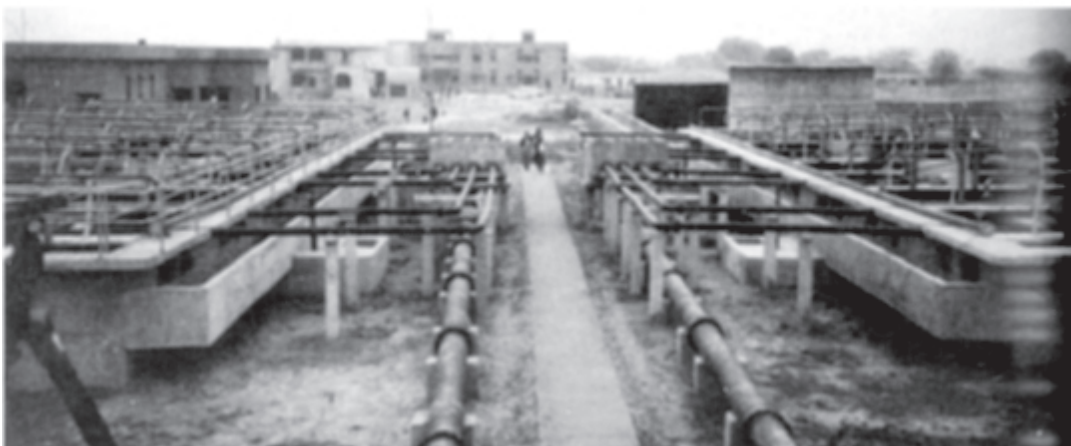
Photo 11.3 45 MLD capacity sewage treatment plant under Yamuna Action Plan at Faridabad, Haryana Source MoEF Annual report 1997-98
