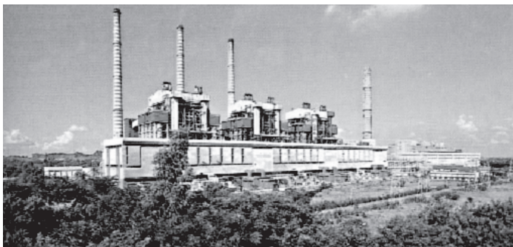
Photo 3.2 Ramagundam super thermal power project Source Ministry of Power, Annual report 1999-2000
