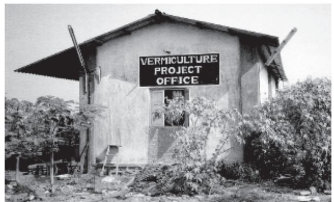
Photo 12.4 Vermi Compost plant for treatment of solid waste
