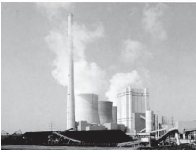
Photo 2.3 Thermal power generation
