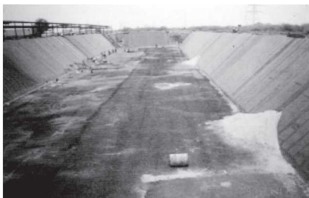
Photo 12.1 Secured landfill for disposal of hazardous waste under construction
