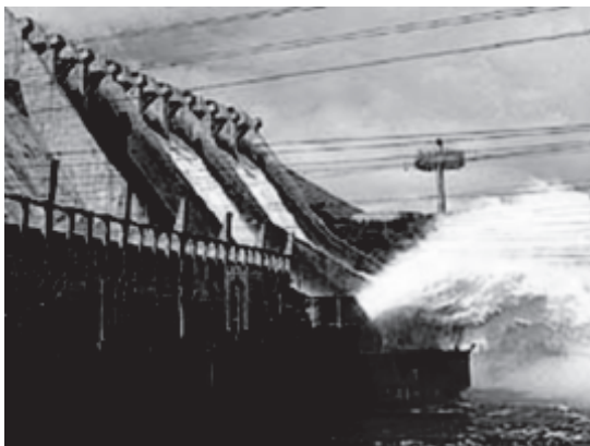
Photo 2.4 Hydro power generation
