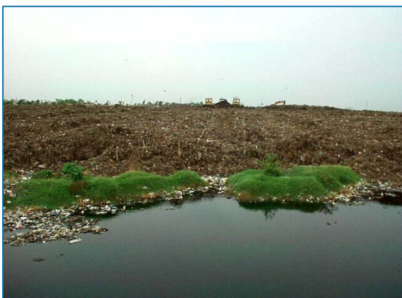
Photo - 3.17. Matuail landfill site (open and without leachate treatment technology)
