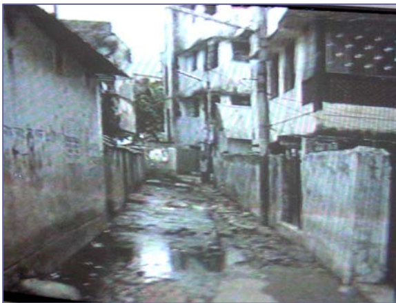
Photo - 3.23. Sewage overflow in old Dhaka
