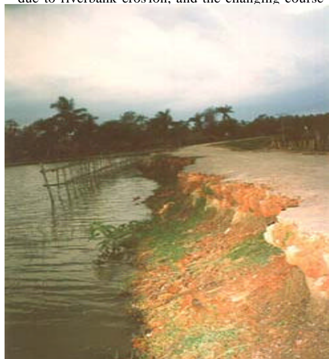
River bank erosion
