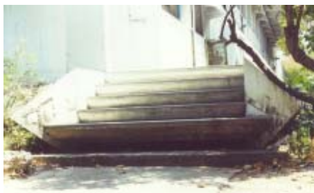
Figure 5.1 Land subsidence causes damage to the several building and infrastructure in Bangkok
