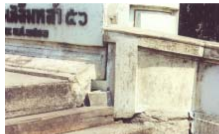
Figure 5.1 Land subsidence causes damage to the several building and infrastructure in Bangkok
