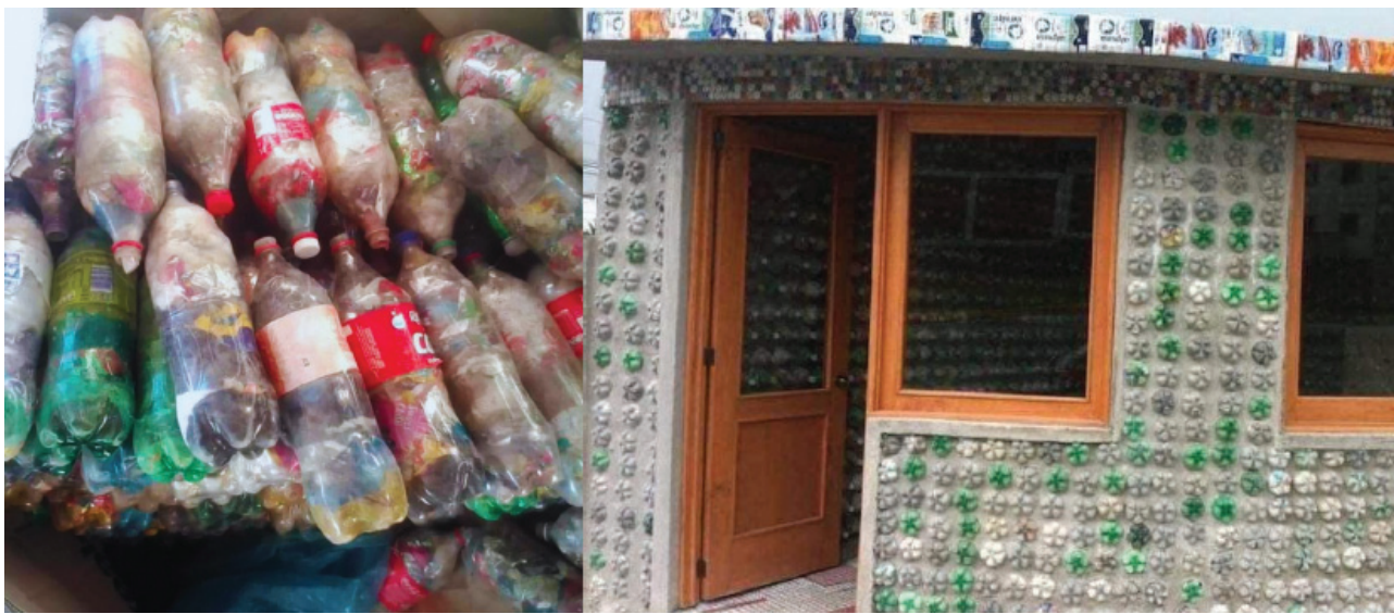
Iloilo City showcase an ECO Brick, a project of St. Therese MTC Colleges to build housing units using ECO Bricks.
