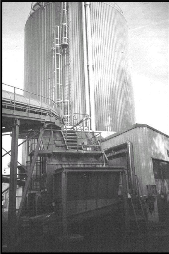
Figure C-11 Example of high-solids anaerobic digester
