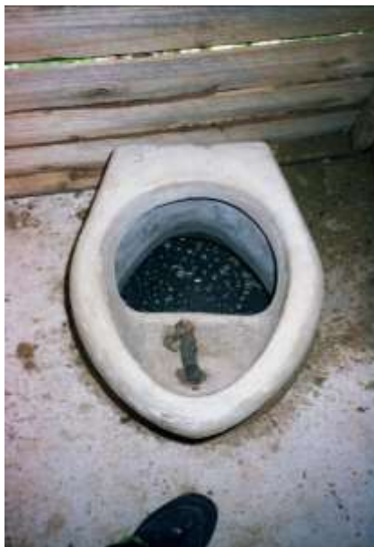
Fig 3.1. Fecal cross contamination to the urine constitutes the major health risk in the subsequent handling of this fraction. It is necessary the toilets to be adapted to the user and the system.
