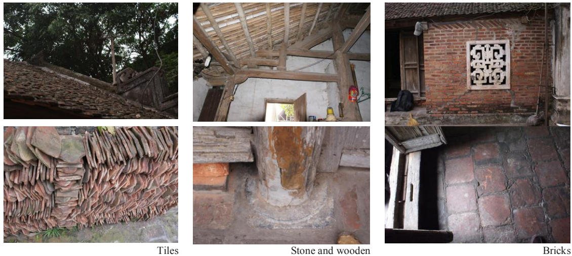
Fig. 13. Materials in Traditional rural house in the Northern lowland (Owner: Le Huu Di, Ngoc Loi, Ngoc Tu, Bac Ninh)
