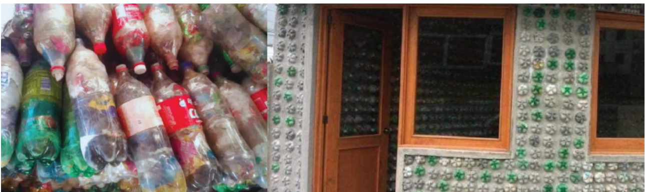
Iloilo City showcase an ECO Brick, a project of St. Therese MTC Colleges to build housing units using ECO Bricks.
